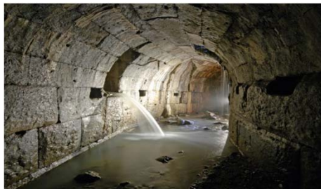
Sewers/drains: Cloaca Maxima
