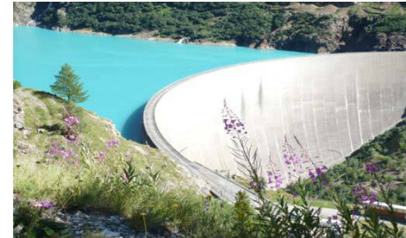
Water reservoir for security of supply
