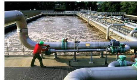
Wastewater treatment plant
