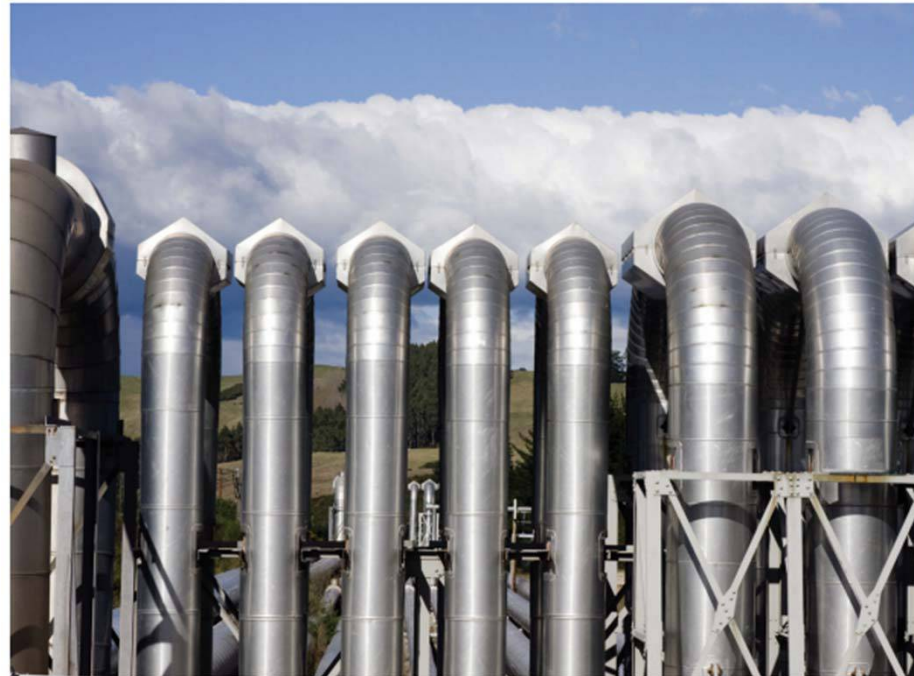
© Jimmy Lopes | Dreamstime.com - Geothermal Power Plant Producing Alternative Green Energy.
